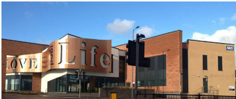
Figure 3: Kensington Neighbourhood Health Centre (Source: Maliene, 2014)
