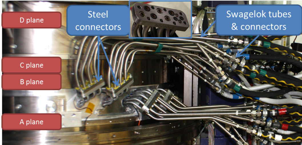
Figure 4.22: Heat transfer platform installed in LISA and connected to the water network.
