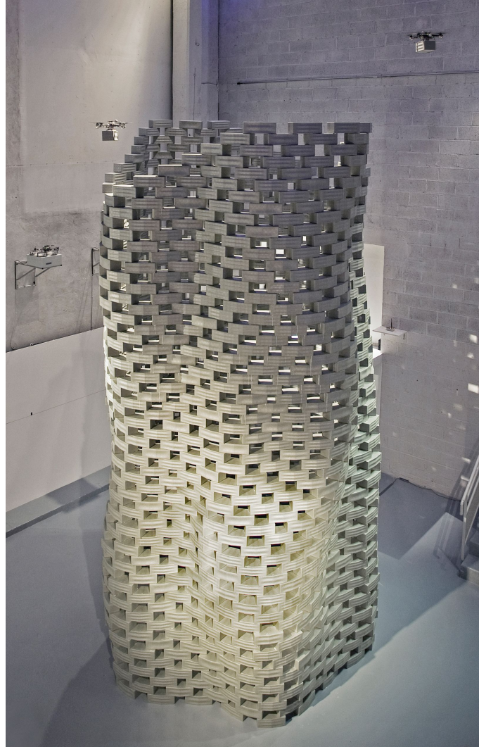
Figure 10. Tower made of foam bricks, assembled by quadrocopters during the Flight Assembled Architecture project [41]. Two of the quadrocopters can be seen above the tower to the left and right; a third is seen resting on a charging station on the wall to the left. The flight paths used by the quadrocopters for this project were generated using the trajectory generation algorithm presented in this paper.
