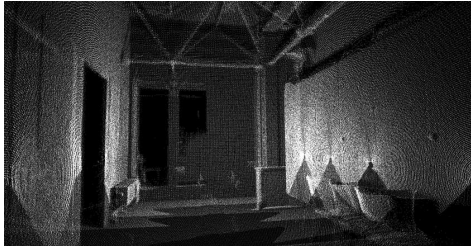
(a) A point cloud based on registered scans showing a part of a corridor.
