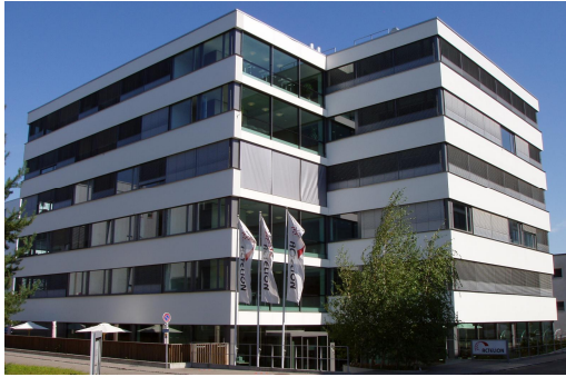
Fig. 1 The demonstrator building (view from South).
