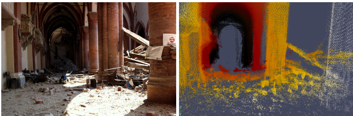
Figure 5.6: Comparison of the point cloud reconstruction with a photograph taken during exploration. Left: Photograph of the western gallery with the collapse roof on the right. Right: Front view of the reconstruction.
