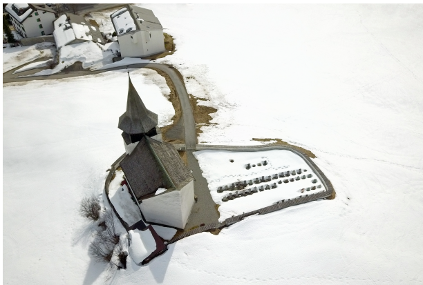
(a) The church in Davos Frauenkirch was rebuilt with a wedge in 1602, intended to deviate future avalanches past the building on both sides. The modern building (background right) is situated in the blue zone and has a reinforced concrete wall in upstream direction without (large) openings (photo: E. Hafner).
