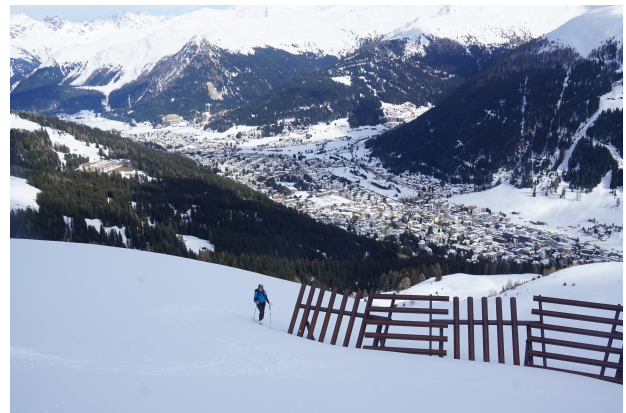
(b) Steel supporting structures at the Grüniberg stabilizing the snowpack and preventing avalanches from starting in the release area, thereby protecting the city of Davos beneath. The structures are dimensioned according to the expected snow heights, since snowed-in structures lose their protective function (photo: I. Rittmeyer).
