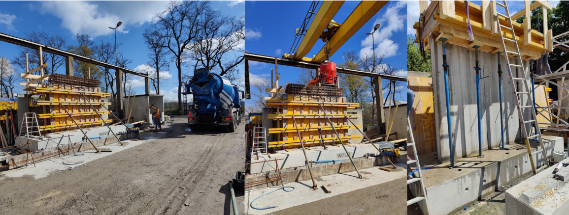
Figure 3.5: Wall framework and concrete casting.
