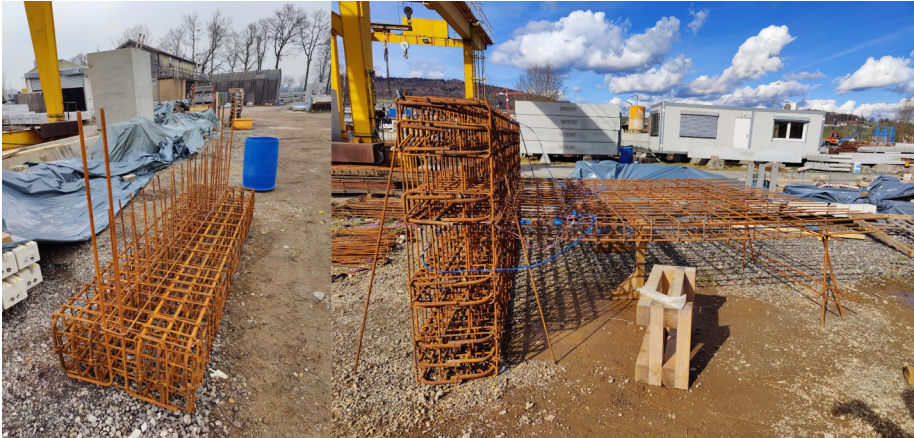
Figure 3.3: Assembled steel reinforcement.
