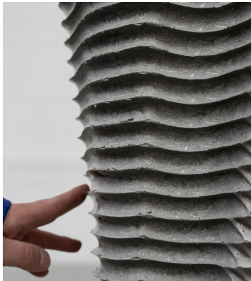
Figure C.3: Close-up of sharp concrete details.
