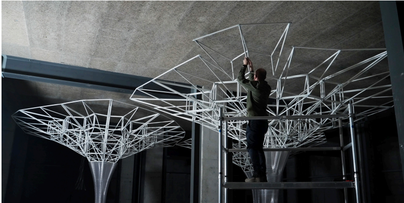
Figure 6.11: Supportfree assembly, last element being placed. Photo: Girts Ap-skalns, girtsapskalns.com.
