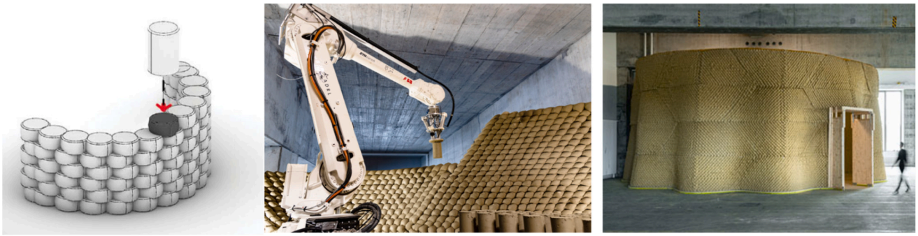
Fig. 3. Scheme illustrating the operation of the discrete deposition method (adapted from [58]) (left) employed in the construction of the Clay Rotunda by Gramazio Kohler Research, in collaboration [56] (middle and right).
