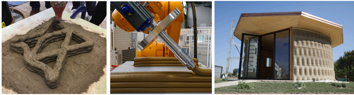
Fig. 2. Robotic 3DP cob with wheat straw by [54] (left), 3DP earth based material with alginate as a bio-stabilizer by [30] (middle) and Gaia Project (right) first large scale earth printed house [55].
