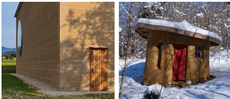
Fig. 1. Prefabricated Rammed earth wall for Ricola Kräuterzentrum by Herzog & de Meuron with Martin Rauch [47] (left) and an example of a Cob house construction [48] (right).
