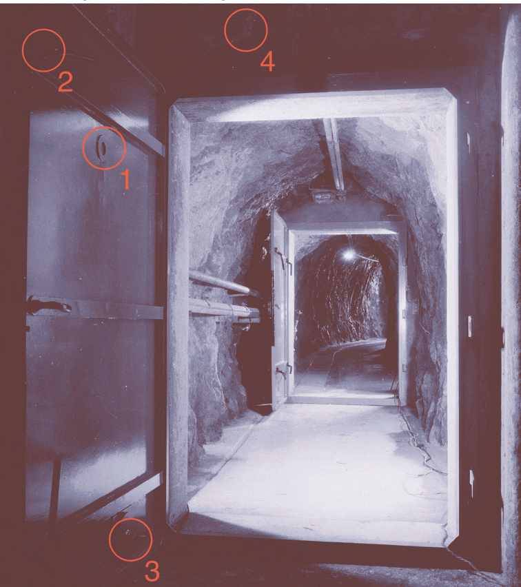
Figure 6 Photograph of armored doors inside the K8 bunker, annotated with evidence 1, 2, 3, and 4
