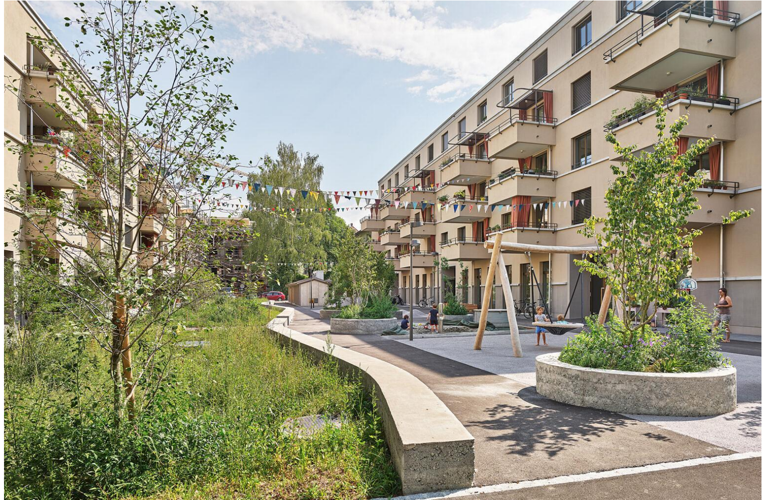
Bern, Wylerhof. Utilisation density of 241 inhabitants and employees per ha ( Fluri, Miriam, W2H Architekten )
