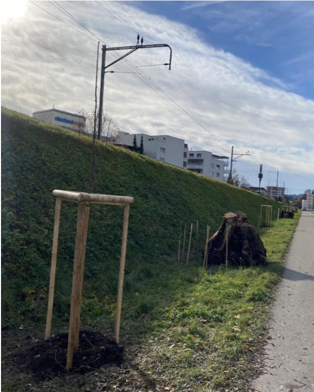
Slow Mode Axis along the train dam at Färberwiese (own picture)
