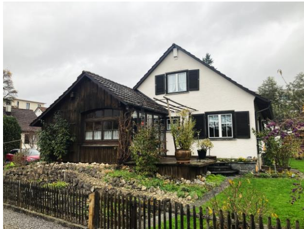
Example for building structure (own picture)
