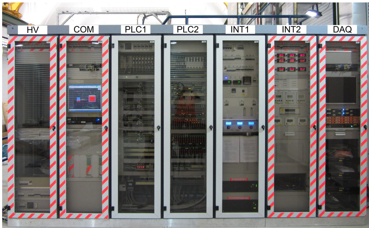
Figure 4.1: The seven standard 19" racks containing the ArDM control system (COM, PLC1, PLC2, INT1 and INT2 rack), the high voltage supply of the PMTs (HV rack) and the data acquisition system (DAQ rack).
