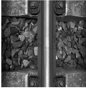
(a) Healthy weld (camera mounted on a diagnostic vehicle of the SBB).
