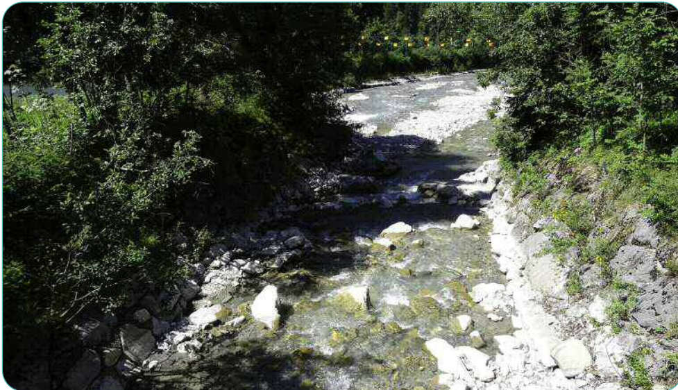
Fig. 05: Well-designed riprap can help shrub vegetation to grow (Big trees can cause riprap to collapse and must be removed). Eric Bardou, UNHCR 2022.
