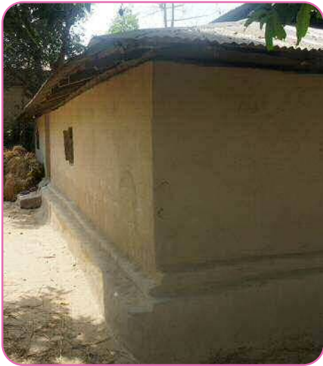
Fig. 11: Traditional house in Bangladesh with a double sacrificial layer. J. Horta, CRAterre, 2018.
