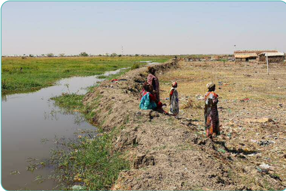
Fig. 04: Example of an earthen dike in the Al-Redis Refugee Settlement. Philippe Reymond, UNHCR 2023.
