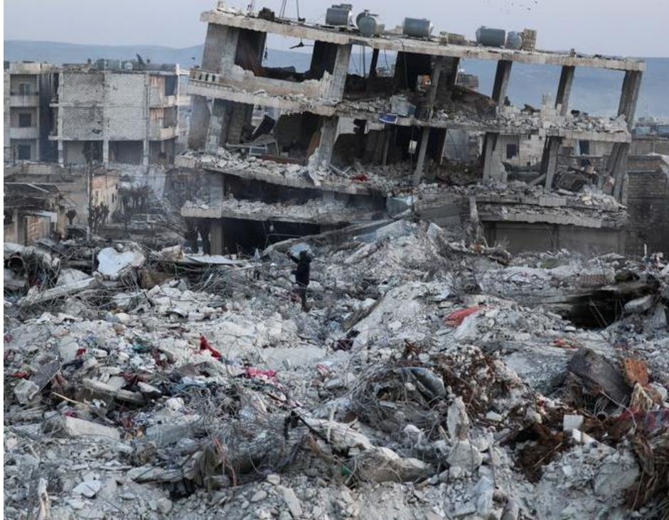
Figure 4.30. Collapsed building (foreground) and a partially collapsed RC building (background) in Jandires, Northern Syria (Source: Reuters ).
