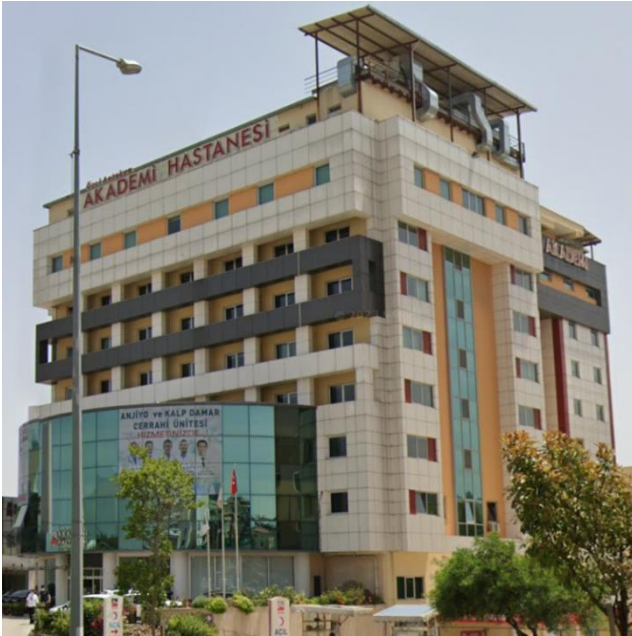
(a) Pre-earthquake view ( Google Maps )
