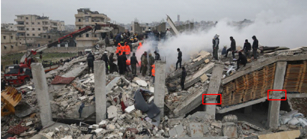
Figure 4.28. Slab failure in a collapsed building in Samada, Northern Syria (Source: https://news.un.org/en/story/2023/02/1133177 ). Notice the complete damage to the slab-column connection in the two right columns.
