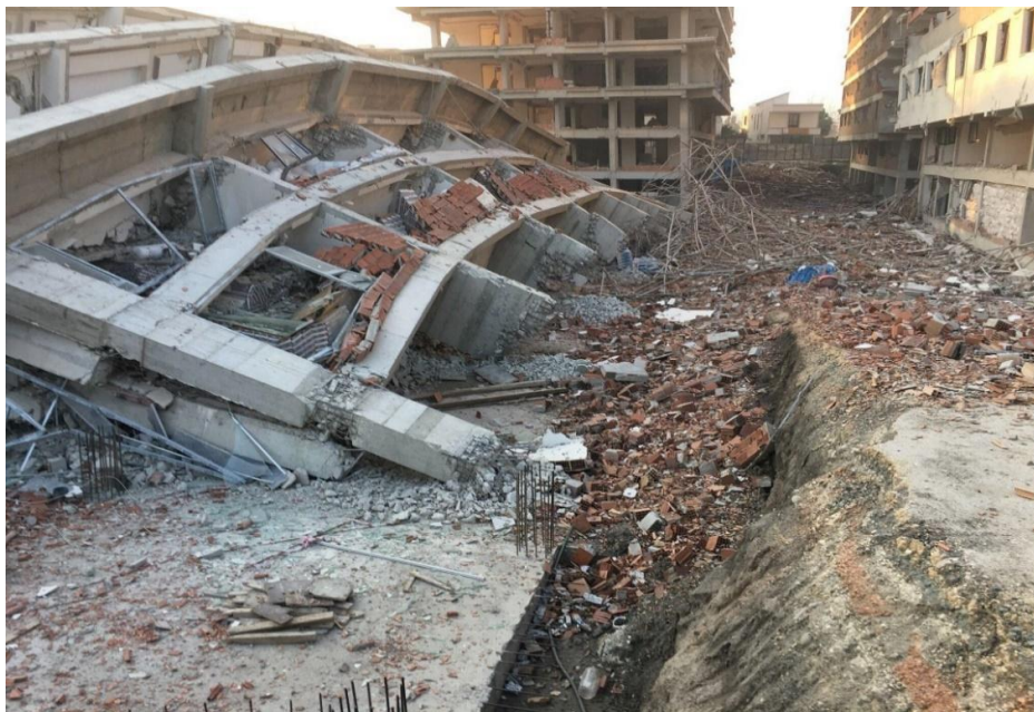
Figure 4.16. Collapse of an RC building under construction (Source: Earthquake Engineering Association Turkey ).
