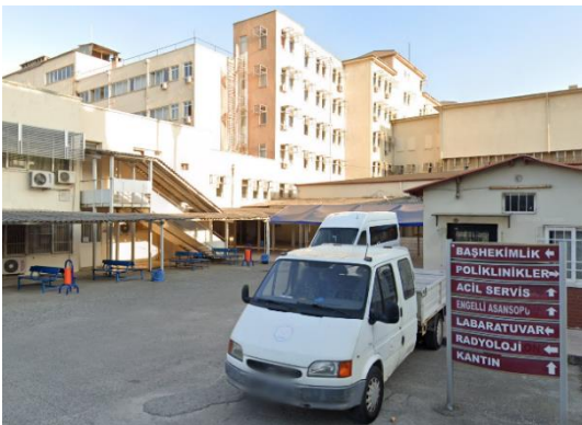
(a) Before the earthquake sequence ( Google Street View ).
