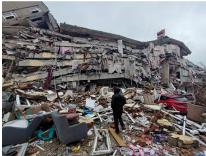
Figure 1.5. Collapsed multi-family residential building in Kahramanmaraş. The photograph illustrates how observed collapse scenarios lead to complete loss of contents and the inability to recover personal possessions (Source: Reuters via CNN ).
