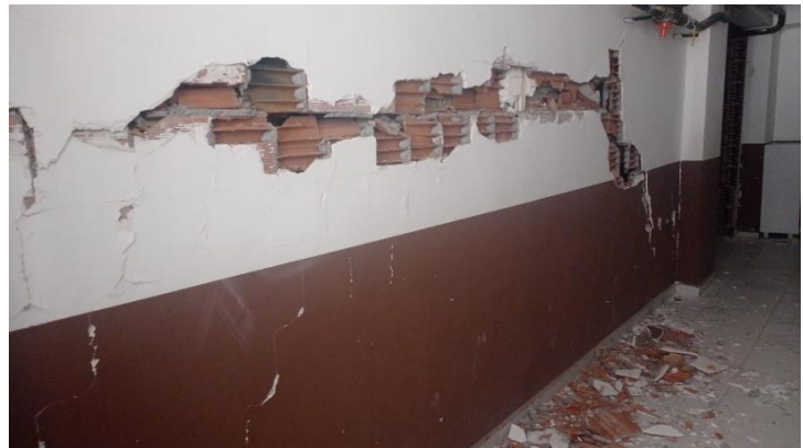
(b) Interior wall.
