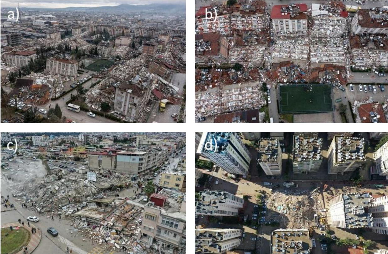
Figure 4.3. Aerial views of the extent of damage in some cities in Türkiye after the earthquakes: a) and b) show mid-rise RC residential buildings that have collapsed in a side-sway manner, while nominally identical buildings in the same developments are damaged but have not collapsed; c) shows two corner RC buildings that have collapsed, possibly due to torsional eccentricity; d) shows a single high-rise building that has collapsed among other similar high-rise buildings that did not collapse (Source: (a) Getty Images via BBC , (b) Independent , (c) Getty Images via CNN , (d) Getty Images via CNN ).
