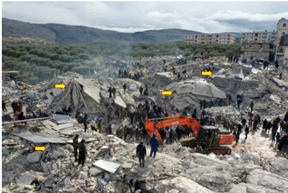
Figure 4.25. Pancaked collapse of masonry and RC buildings (shown with arrows) in Besnaya, Reef Idlib (Source: AFP via npr.org ).
