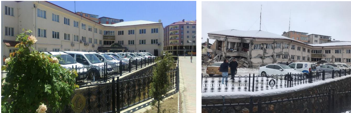
Figure 4.40. Afsin-Kahramanmaraş municipality building before (Source: Google Map ) and after (Source: Twitter ) the earthquake sequence (38.2441N, 36.9151E). The collapse of one wing of this building with an L-shape plan might be due to torsional effects and plan irregularity.
