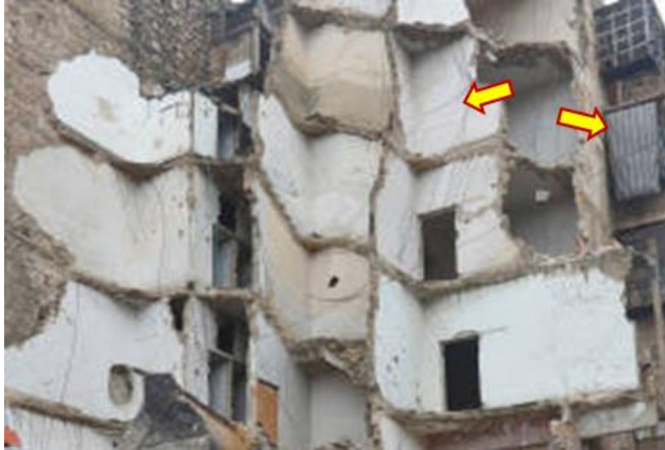
Figure 4.23. Ruins of a collapsed masonry building in Aleppo (Source: LOUAI BESHARA/AFP, Getty Images ).
