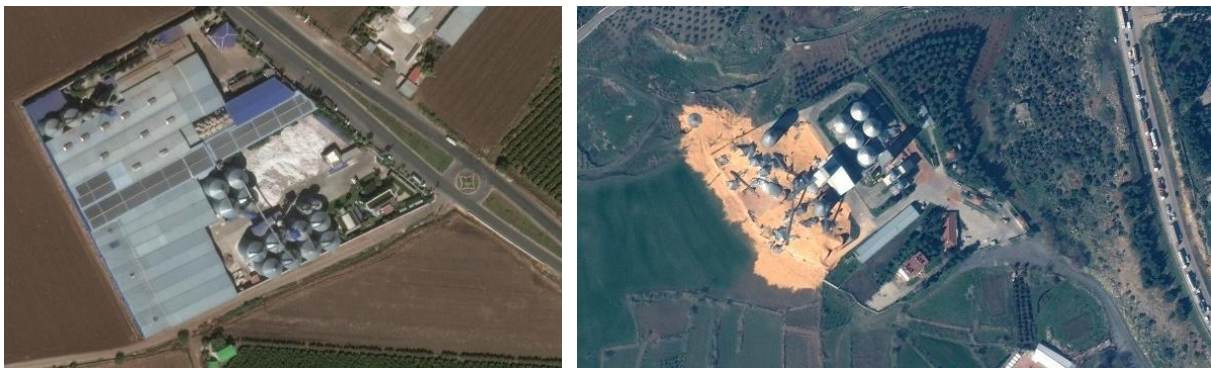
Figure 5.12. Aerial views of the damage of grain silos near Kırıkhan (Left) and near Nurdağı (Right) (Source: CNN ).
