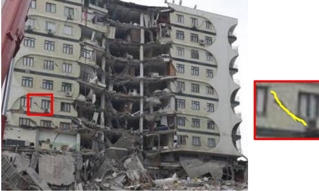
Figure 4.14. Partially collapsed building showing major diagonal cracks (refer to the insert) on the remaining towers, Diyarbakir (Source: Getty Images ).
