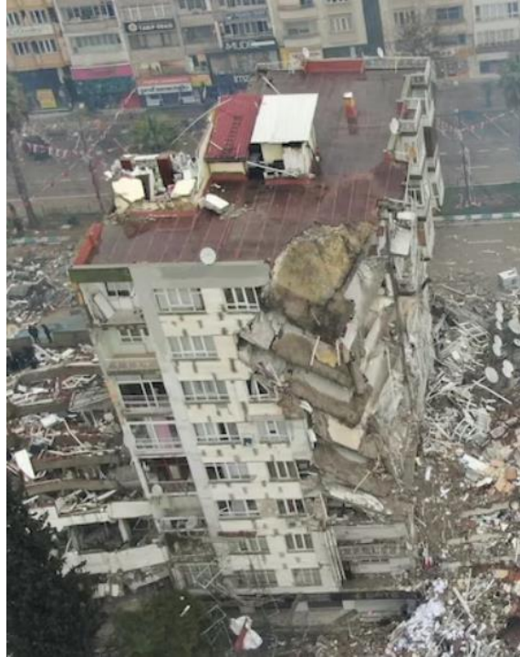
Figure 4.20. Partially collapsed of a multi-story building in Kahramanmaras, February 6 (Source: Ihlas News Agency (IHA) via Reuters 2023a ).
