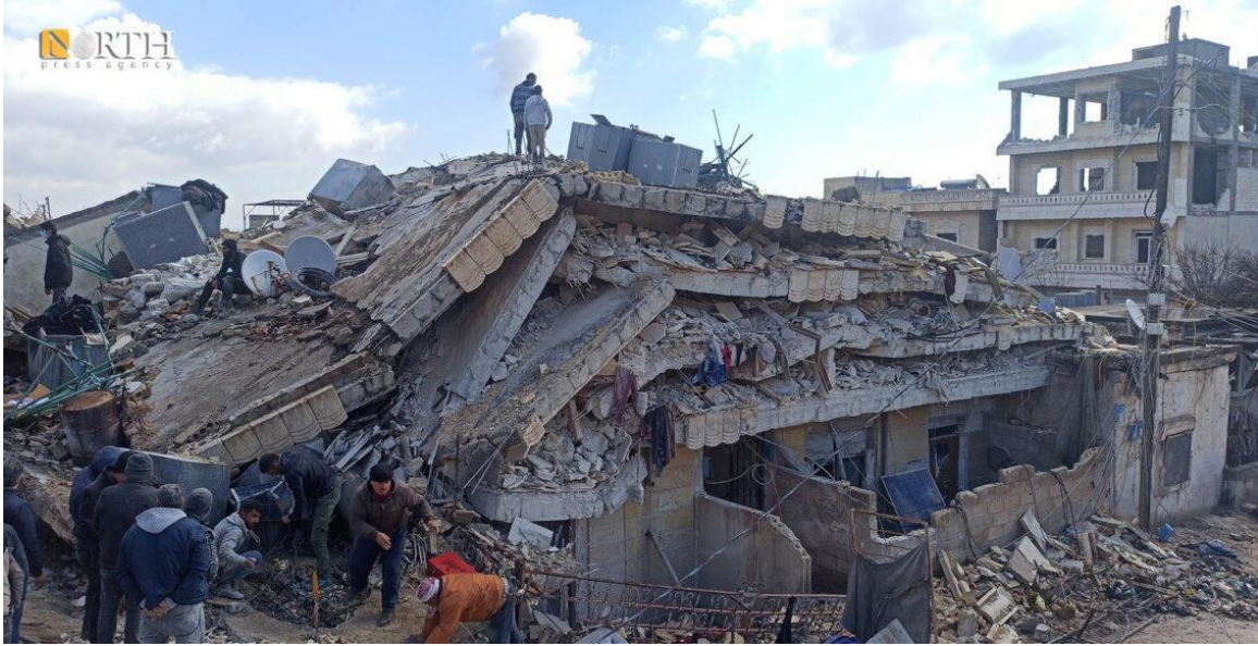
Figure 4.34. Pancaked concrete ribbed slab failure, likely built on unreinforced masonry bearing walls in Jinderis, Northern Syria. Notice the ribbed slab RC construction of the right neighboring building (Source: NPASyria ).
