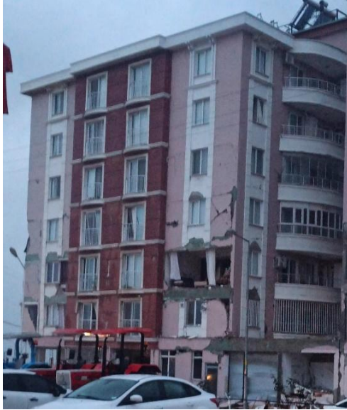
(a) Residents had difficulty exiting the building due to stairwell collapse (Source: Tommy Shelby via Twitter ).
