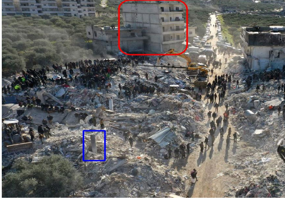
Figure 4.26. Collapsed masonry & RC buildings, Besnaya, Reef Idlib (Source: AFP via npr.org ).
