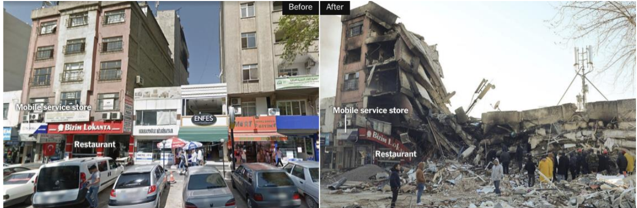
Figure 4.6. Collapse of buildings due to weak/soft story & pounding. The short 2-story building located between two mid-rise buildings, without adequate seismic separation, likely led to pounding between the roof slab of the 2-story building and the mid-height of the adjacent buildings. This has resulted in partial collapse of the building on the left and total collapse of the building on the right along with collapse of the 2-story (Source: New York Times 2023).
