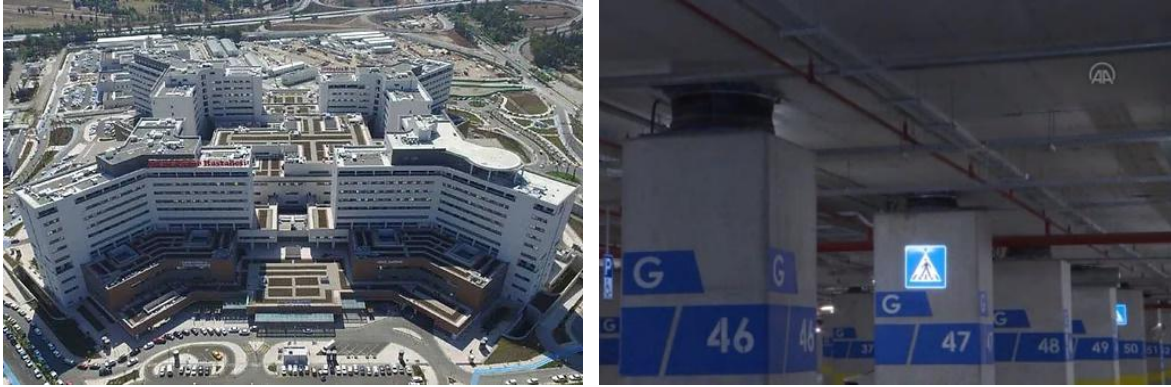
Figure 4.59. Adana City Hospital, 37.0301N 35.3483E (left) (Source: EPS 2023 ) and Frictional pendulum-type base-isolation devices in the hospital building (right) (Source: Anadolu Ajansi 2023 ).
