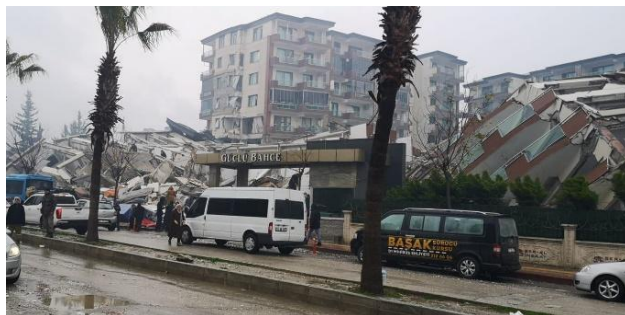
Figure 4.11. Güçlü Bahçe residential building complete collapse in Hatay (Source: Twitter ).
