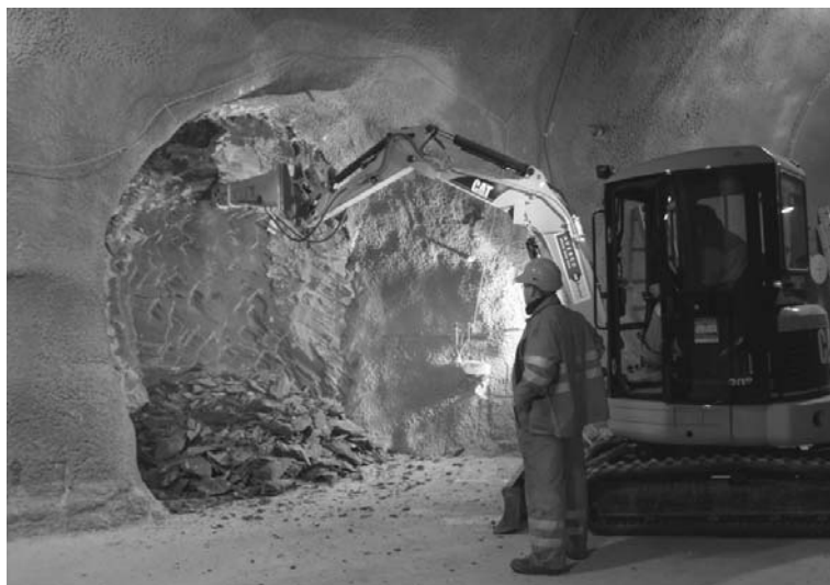
Fig. 5.14: Excavation of the “Mini niche” in the centre of the entrance face.
