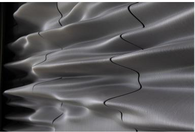
Figure F.9: Close up of the acoustic diffusor panel.
