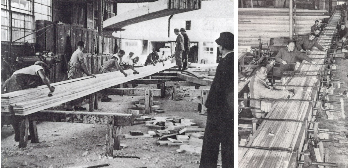
Figs 15-16 Processes of gluing and laminating. The workers, due to the nature of the work, need to perform all the same task, at the same time and with the same speed.
