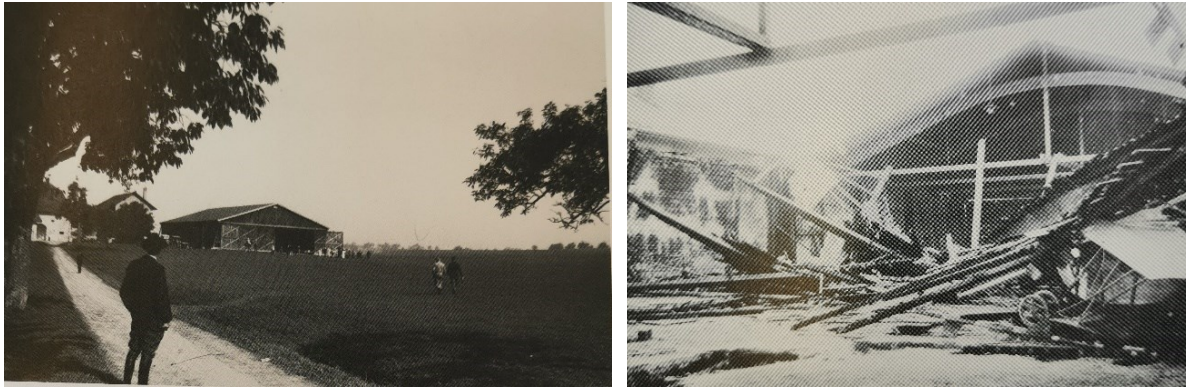
Fig. 4 hangars for the aeroplanes in Blécherette near Lausanne, constructed in 1914. Contractor: Ed. Bugnion.
