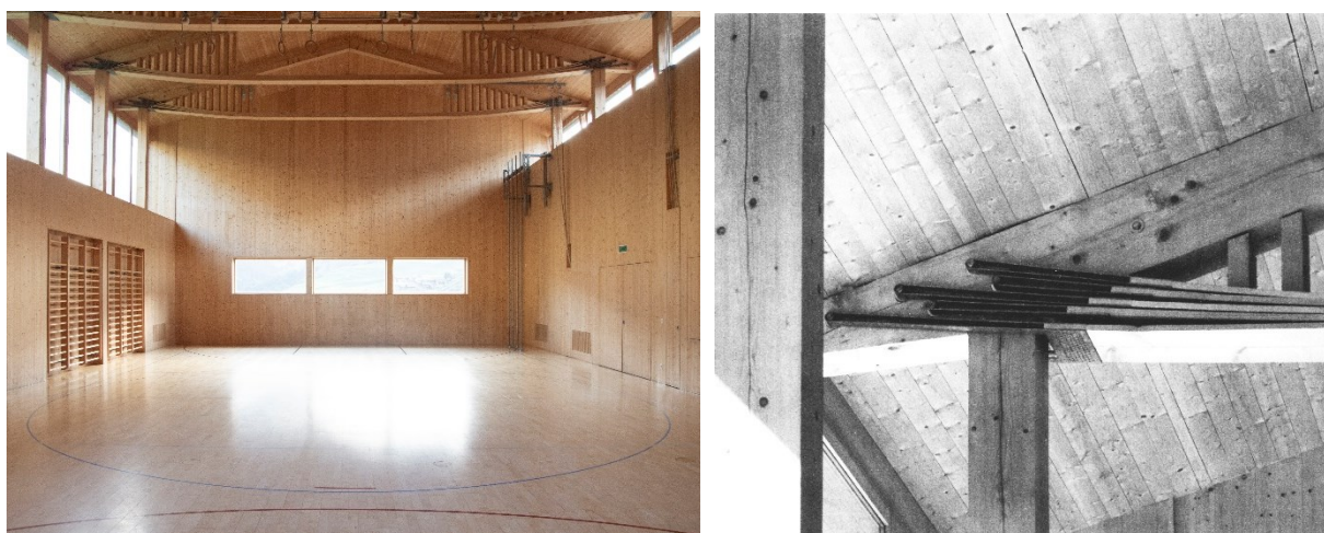
Figs 8-9 Gion Caminada and Jürg Conzett, gym building in Vrin, Switzerland, 1996.
