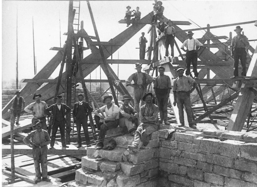
Fig. 45 Carpenters on the construction site of the catholic church in Romanshorn, 1911
