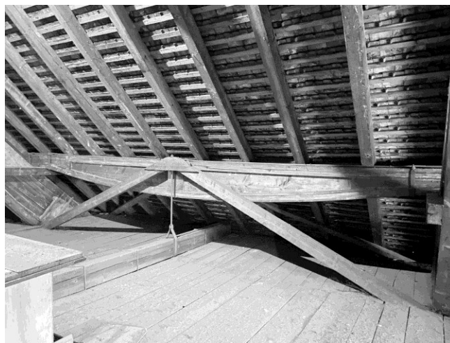
Fig. 29 Sports hall Birsfelden, detail of the purlin, 2019.
