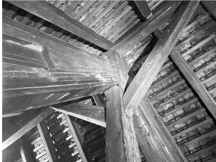
Fig. 30 Sports hall Birsfelden, detail of the hanging post and rafter top, 2019.
