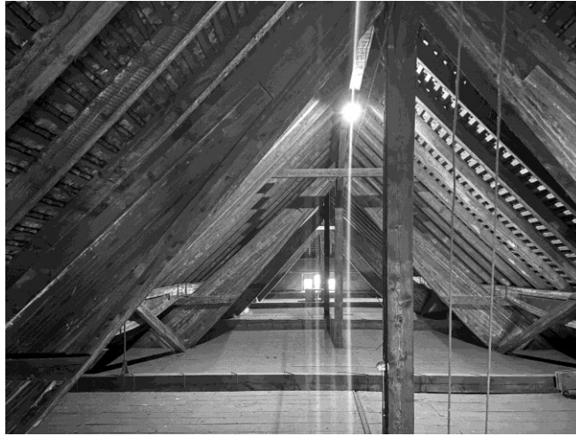
Fig. 28 Sports hall Birsfelden, view into the roof, 2019.
