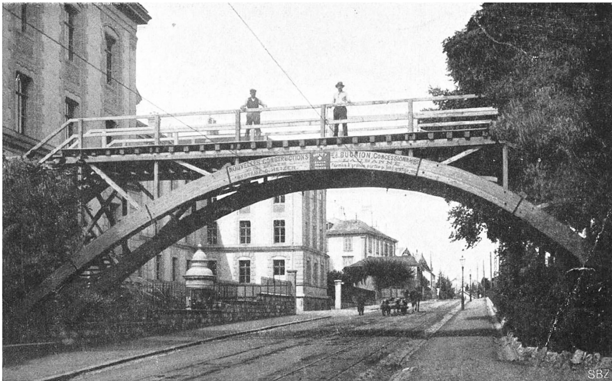
Fig. 6 Glulam pedestrian bridge on the occasion of the 8th National Exhibition of Agriculture, Lausanne, 1910. contractor: Ed. Bugnion.
