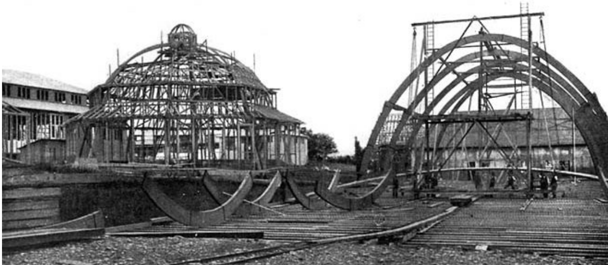
Fig. 5 Construction site of the pavilion for the Building Industry. Bern, 1913. At left, the glulam structure is getting assembled and erected.
