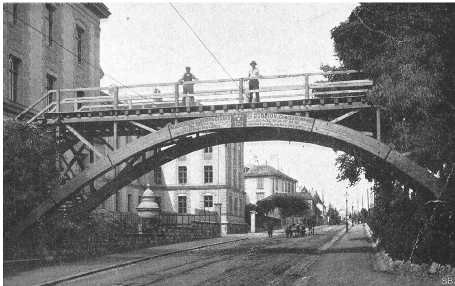
Figs 46-47 Temporary glulam bridge at the 8th Swiss Exposition of Agriculture, Lausanne. contractor: Ed. Bugnion, 1910.
