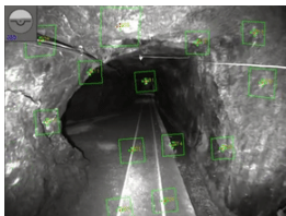
(a) Visual-inertial odometry in difficult conditions, in an underground mine, using ROVIO [5].
