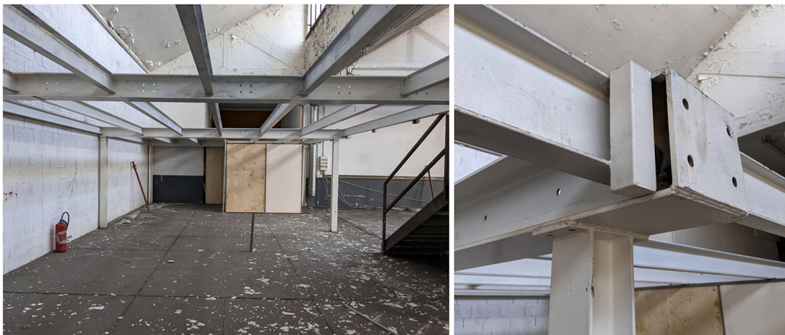
Fig. 2. Overview of test location (left), typical connection at location (right).
