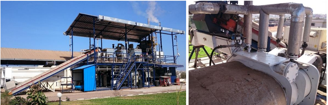
Figure 3.16. Left: a contact dryer at the Omni-processor pilot plant at Niayes FSTP in Dakar, Senegal. In this plant, the sludge is incinerated leading to the generation of heat and electricity. Right: part of the heat from combustion is recirculated in the process for the drying of the sludge with this contact dryer unit (photos: UKZN PRG).
