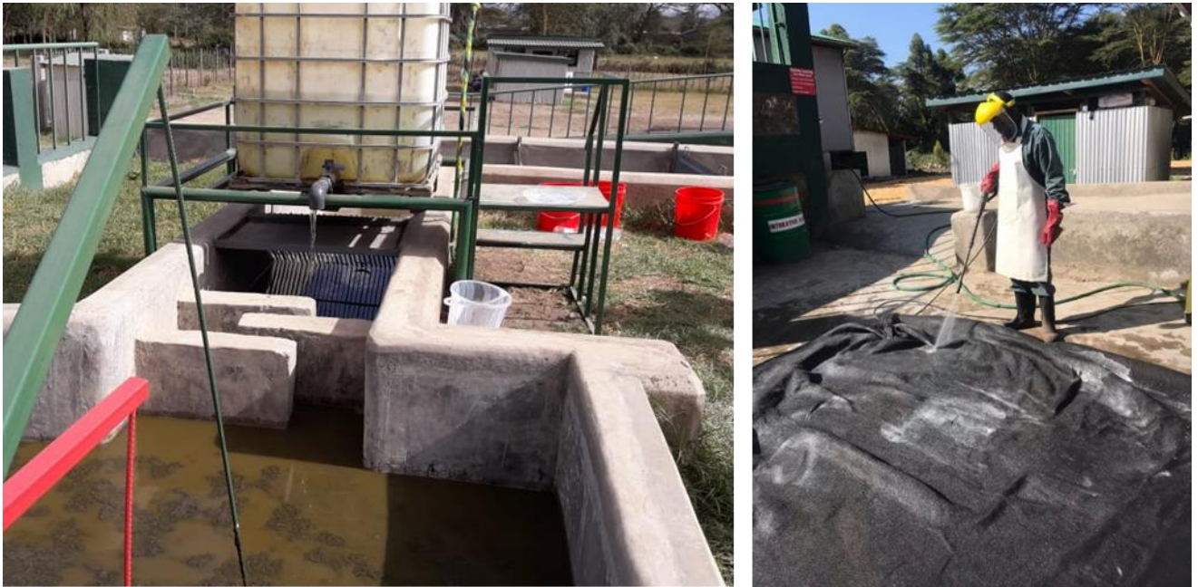
Figure 3.12. Left: an example of a conditioner dosing configuration: one dosing port followed by mixing with baffles and right: a Sanivation employee washes detergent, salt, and particulate residue from a geotextile using a high-pressure water rinse (photos: Sanivation).
