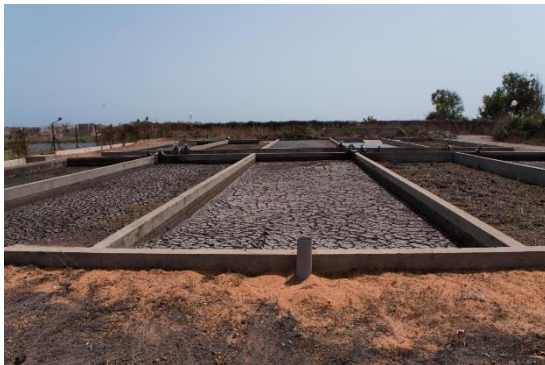
Figure 3.3. Drying beds at Niayes FSTP, Dakar, Senegal (photo: Sandec).
