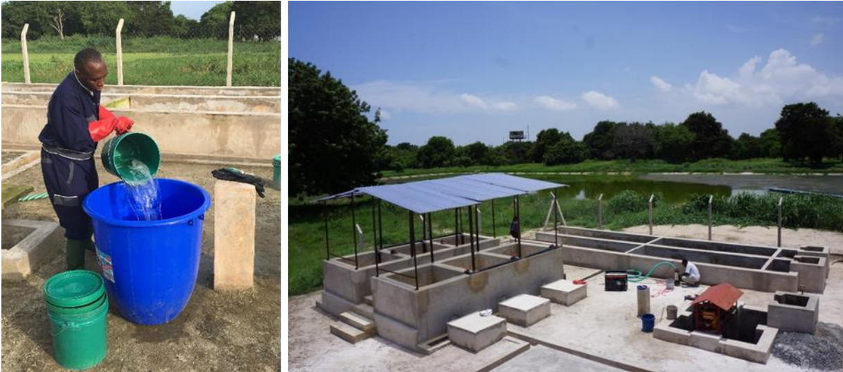
Figure 3.9. Left: mixing chitosan conditioner for pilot-scale trials. Right: the pilot-scale dewatering research facility at the University of Dar es Salaam, including the settling-thickening tanks, conditioner mixing tank, and six sand drying beds (photos: Sandec).
