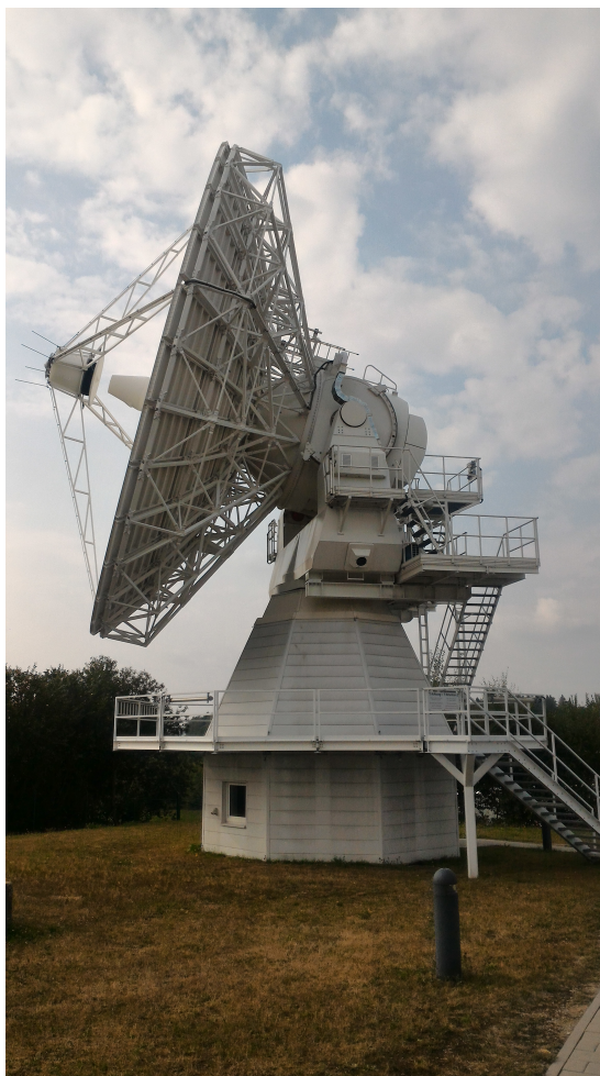
Figure 2.2: WETTZ13S VGOS Antenna in Germany
