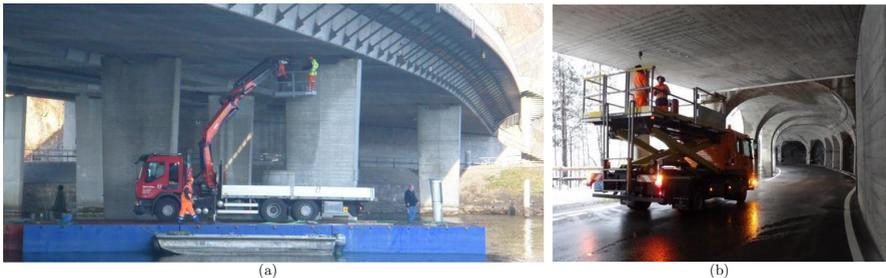
**Figure 1.7:** Challenges in traditional bridge inspection: (a) a floating platform is used to support a truck inspecting the underside of a bridge, and (b) an inspection truck with a lifting platform requires lane closure and frequent repositioning, while workers lift inspection equipment repeatedly above their heads for the duration of the work.
