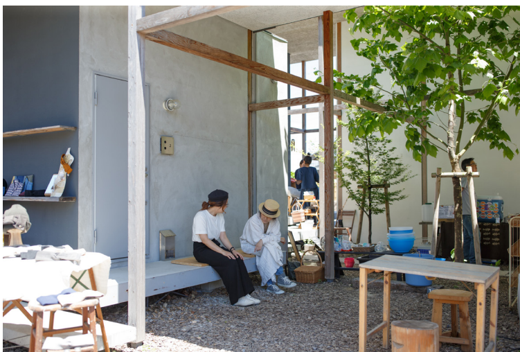
Fig 6 A project that elucidates Satoshi Sano’s interests in developing new forms of (suburban) shared living is Dragon Court Village (2014), an apartment building for 9 families in which exposed structural wooden frames also function as exterior furniture as a means to connect residential life to the community.
