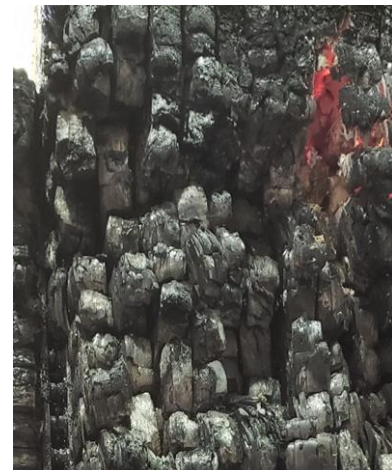
Figure 6: Glowing combustion within the char layer on a glulam column (600 mm x 600 mm) after a standard fire test of 120 min (prior extinguishment)
