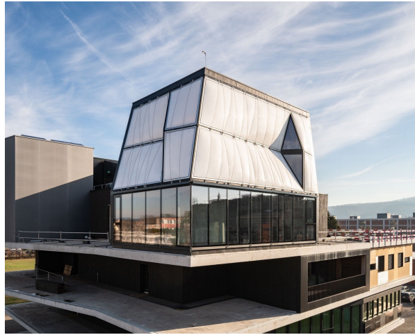
Figure 5.3: DFAB HOUSE at NEST at Empa in Switzerland. Copyright: Roman Keller.
