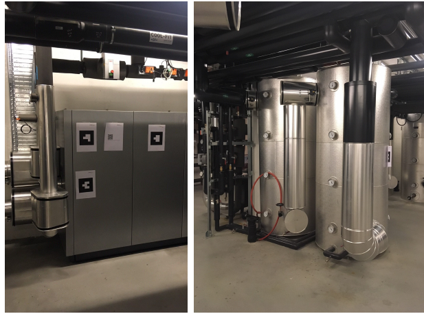
Figure 3.4: Experimental facility with heat pump (left) and water storage tanks (right) (Bünning et al., 2020c).
