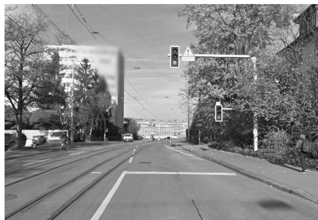
Figure 10. Traffic signal to provide public transport priority at end of a dedicated tram lane. Source: Google Maps.
