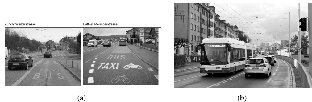
Figure 9. Special dedicated bus lanes: When the flow of buses is too low or in order to also provide priority to different modes, other types of vehicles are allowed (taxis, bicycles, etc.). Similarly, there are bidirectional bus lanes that can be used by buses traveling in both directions. Sources: Google Maps and [74] (a) dedicated bus lanes accessible to other selected transport modes and (b) bidirectional bus lane.
