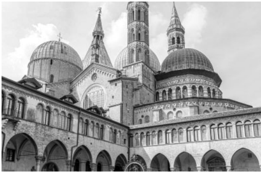
Figure 2. Basilica of St Anthony, south-eastern view (photo: author).
