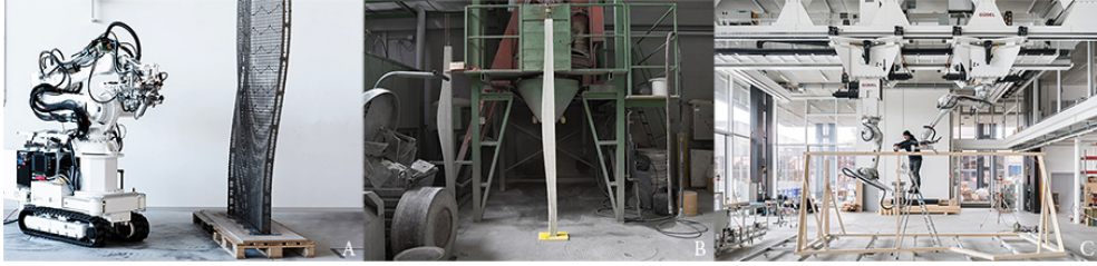
FIGURE 1.3: Three examples of digital fabrication technologies developed and applied in the DFAB House project: A. In Situ Fabricator; B. Smart Dynamic Casting; C. Spatial Timber Assemblies.
