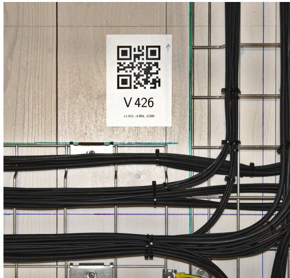
Figure C.1: QR codes used to identify the vertices.
