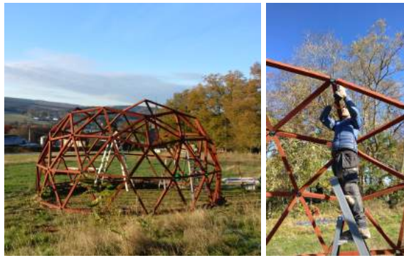
Fig. 1 A geodesic dome example built with renewable materials (Credit: N. Petit-Barreau, Anku).
