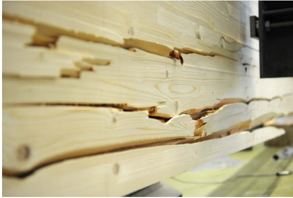
(a) front side ( l \approx 6.3 - 8.5 m), upper crack from 2nd failure cycle
