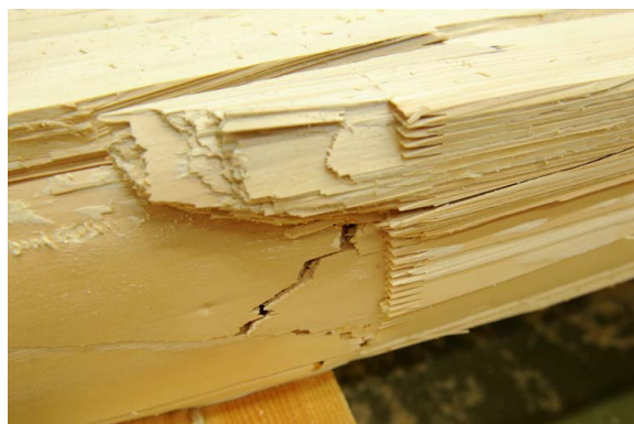
(h) 4th lowest lamella ( l \approx 3.2 m), partly from 2nd failure cycle
