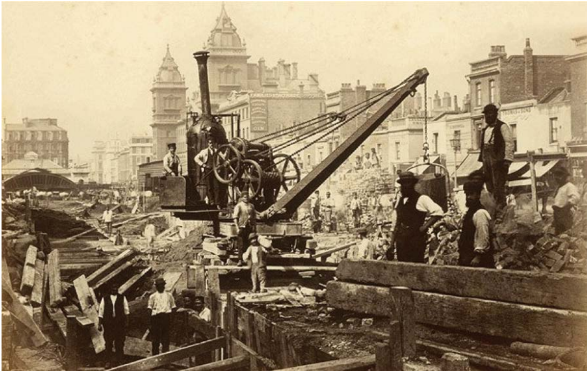
Figure 4. Capitalism meets the city: 1867 photograph by Henry Flather of the construction of the Metropolitan Line at Praed Street next to Paddington Station, forming part of London's new underground railway network (© Museum of London).
