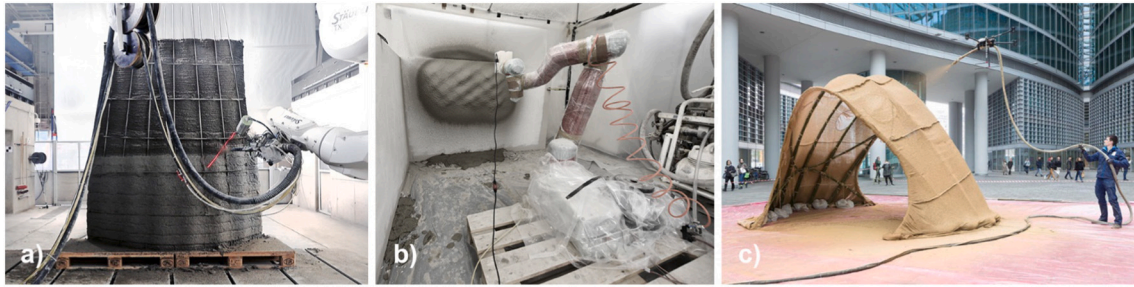
Fig. 5. Spray-based 3DP examples. a) SC3DP of reinforced concrete components [138], b) robotic additive plaster spraying [142], c) drone robot spraying for earthen monolithic shells [141].
