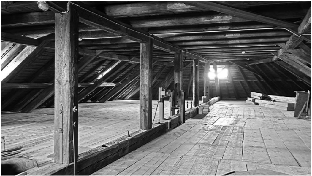
Figure 3. Roof construction of the church (Schäfer 2019).
