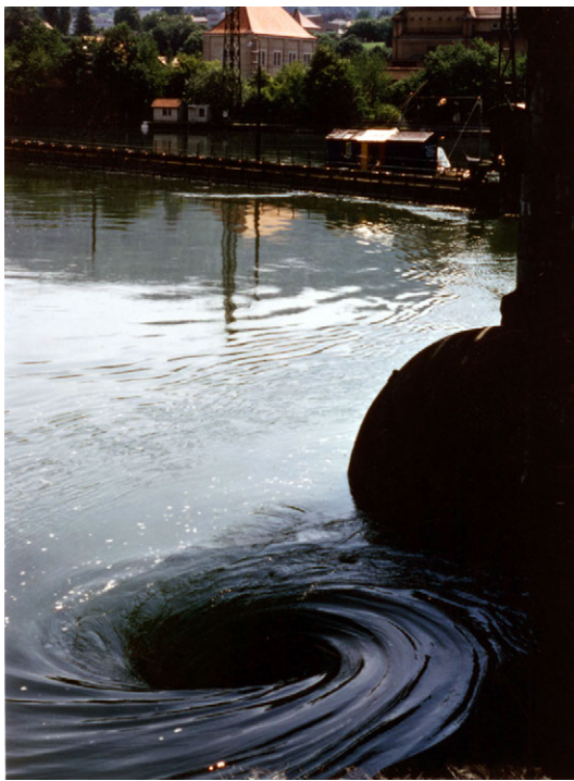
(a) HPP Laufenburg, River Rhine (CH)
