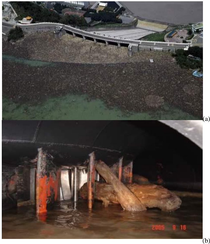
Figure 3: Floating woody debris in Typhoon Aere (a) near dam site (b) turbine clogged by woody debris
