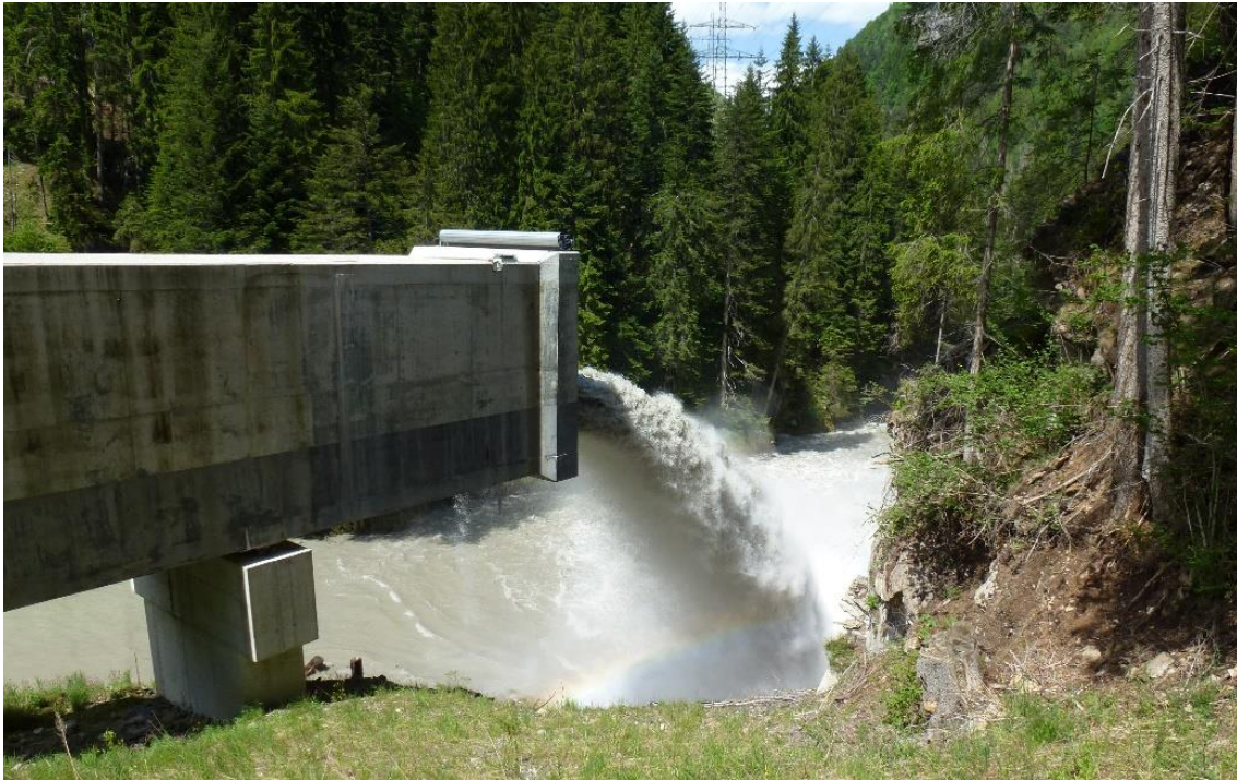
Figure 6: Cantilevering tunnel outlet during operation on May 23 rd 2014 (courtesy of C. Auel)
