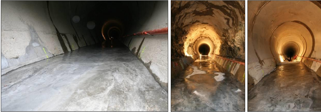
Figure 6: New concrete invert in the most downstream 350 m of the Palagnedra SBT (2013)
