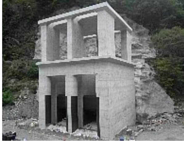
Figure 8: Construction situation of the intake structure
