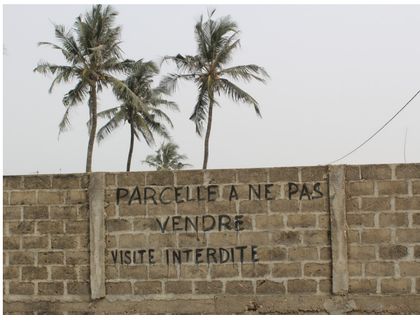
Fig. 66 Construction site of a returnee migrant and retired school teacher in the outskirts of Porto Novo
