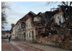
1. Collapsed URM buildings
