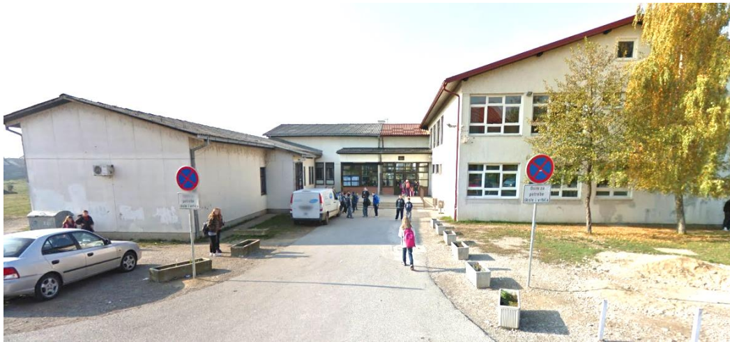
Figure 4.72. Mate Lovraka Elementary School in Petrinja (source: Google Earth).
