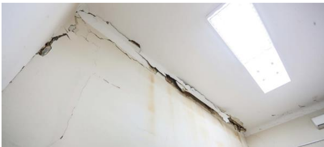
Figure 4.78. Damage at a floor-wall connection at the 2 nd story. The crack at the connection is potentially a result of beam sliding at supports (source https://www.index.hr/vijesti/clanak/video-pogledajte-kako-izgleda-petrinja-ogromna-steta-na-zgradi-gradske-uprave/2242131.aspx ).
