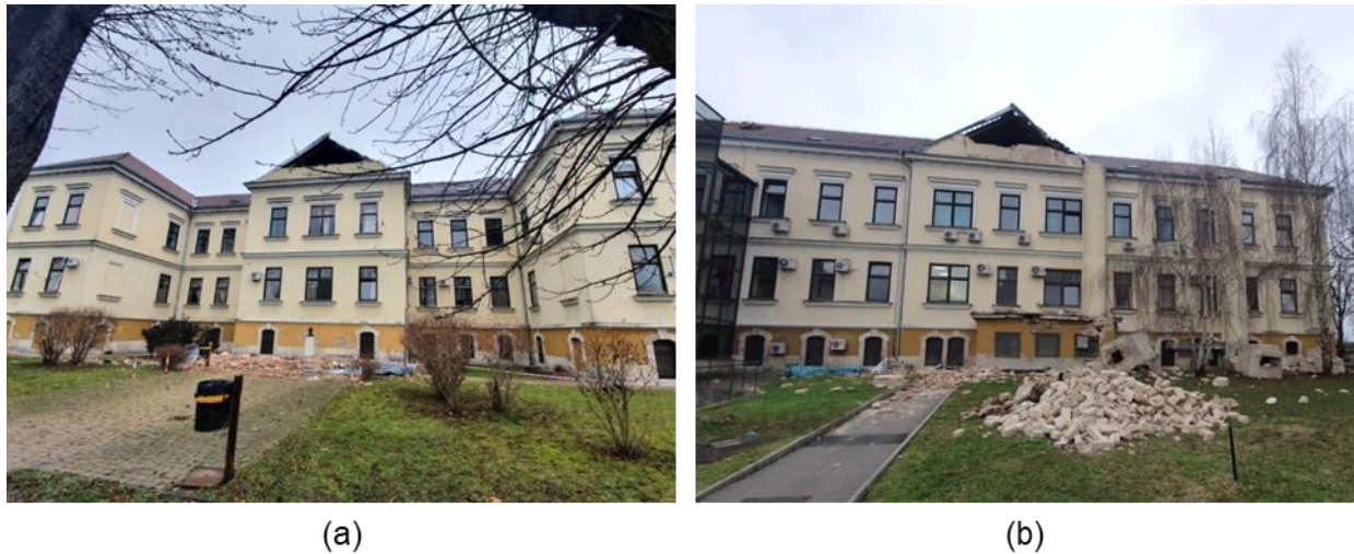
Figure 4.42. Building #2: (a) front view and (b) back view (source: Croatia Week 2021, Jan 5).
