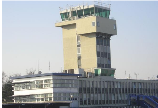
Figure 5.3. Control tower at the Zagreb International Airport experienced minor damage (source: DubrovnikTimes).
