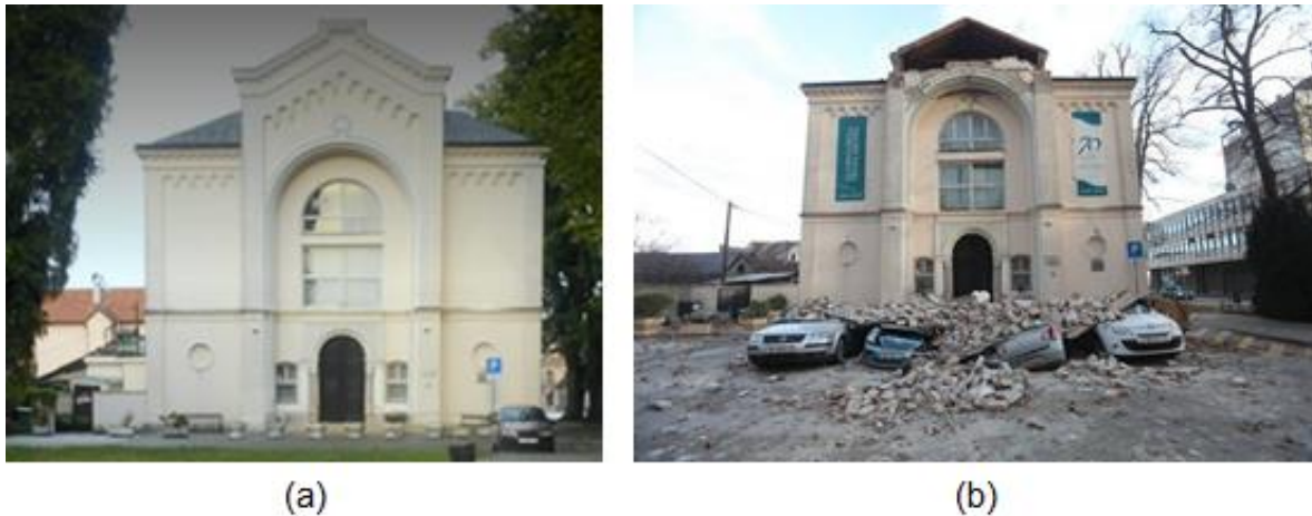
Figure 4.61. Fran Lhotka Music School (a) before the earthquake (source: Google Maps) and (b) after the earthquake (source: Facebook page - Glazbena škola Frana Lhotke, Sisak).
