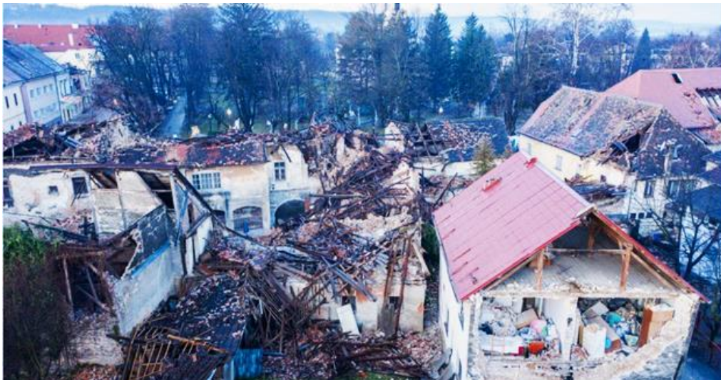
Figure 1.7. Aerial photo showing extent of damage in an area of Petrinja. Photo by Antonio Bronić (Reuters).
