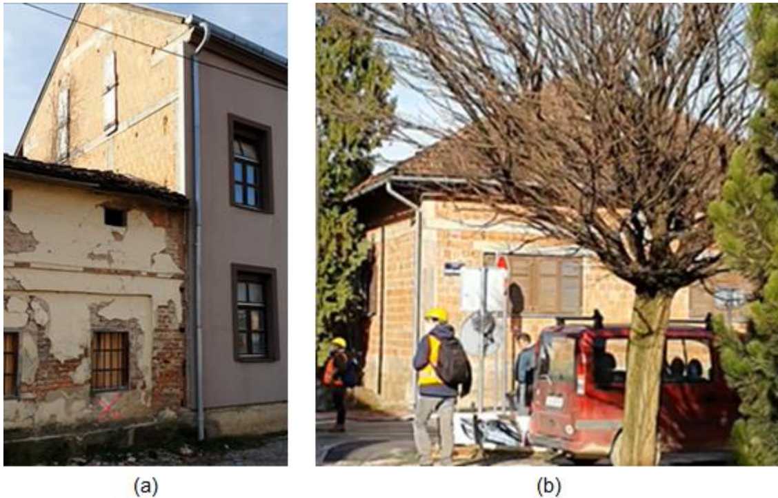
Figure 4.10. Examples of good performance of confined masonry buildings in Petrinja: (a) a two-story confined masonry building remained undamaged while an adjacent older URM building experienced severe damage; and (b) an undamaged single-story confined masonry building (source: Marko Bartolac).
