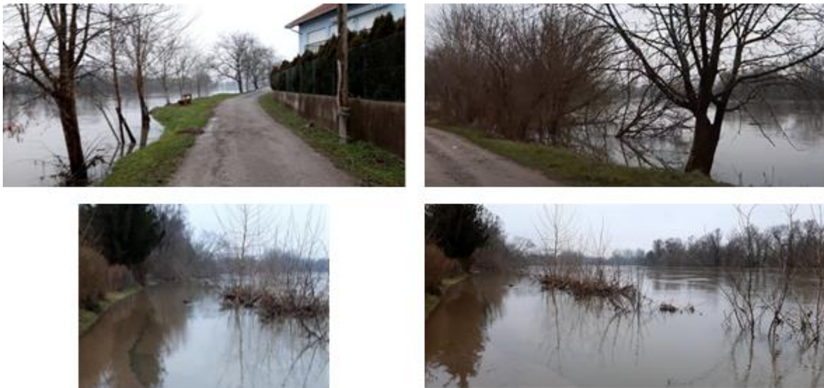
Figure 6.30. Landslide on the coast of the river Kupa, Letovanić (45.5082,16.2118, source Sonja Zlatović).
