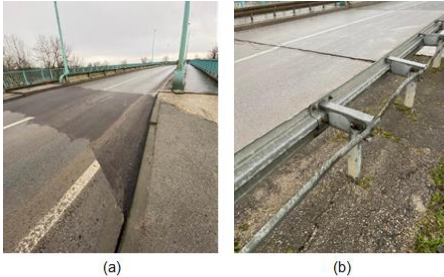
Figure 5.7. Asphalt at right-hand side abutment (a) and asphalt at left-hand side of abutment (b) of the Brest Bridge (source: Mate Baričević).
