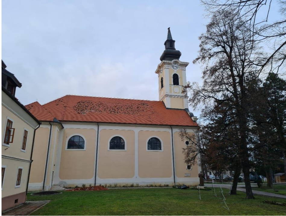
Figure 4.123. Damaged roof tiles on St. Lawrence church (crkva Sv. Lovre) in Petrinja (source: Nenad Bijelić).
