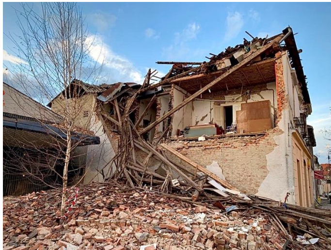
Collapsed unreinforced masonry building on Strossmayer St. in Petrinja, Photo by Damir Lazarević
