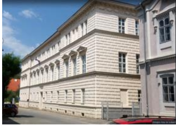
Figure 4.50. Petrinja High School before the earthquake (source: Google Maps).
