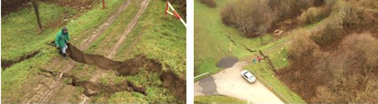
Figure 6.13. Rupture of the left riverbank of Sava (source: Croatian Waters Archive).
