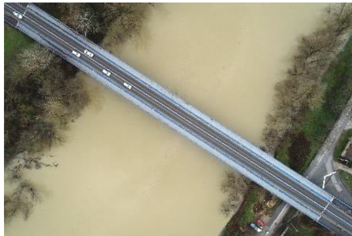
Figure 5.10. Satellite view of Galdovo Bridge (coordinates 45.4791, 16.3848).
