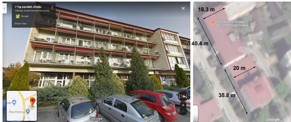
Figure 4.30. Retirement home in Petrinja: outside view (left) and dimensions in plan (right) (source: Google Earth).
