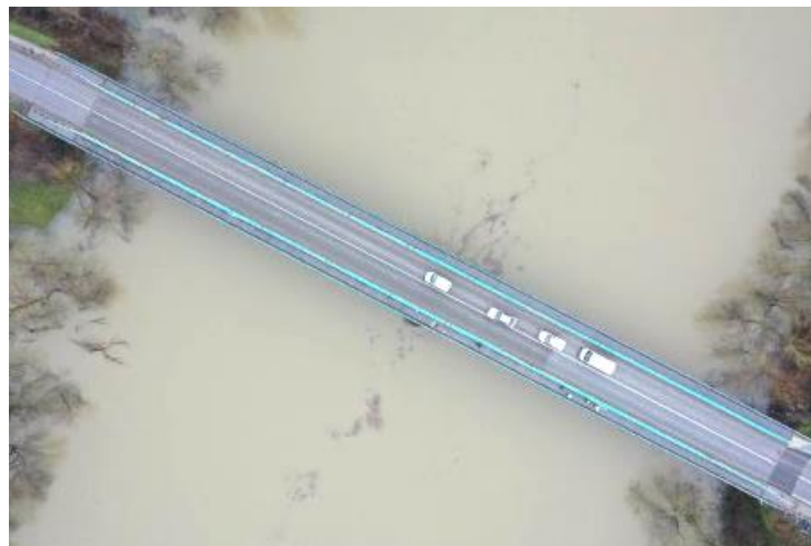
Figure 5.5. Satellite view of the Brest Bridge (coordinates 45.4486, 16.2604).
