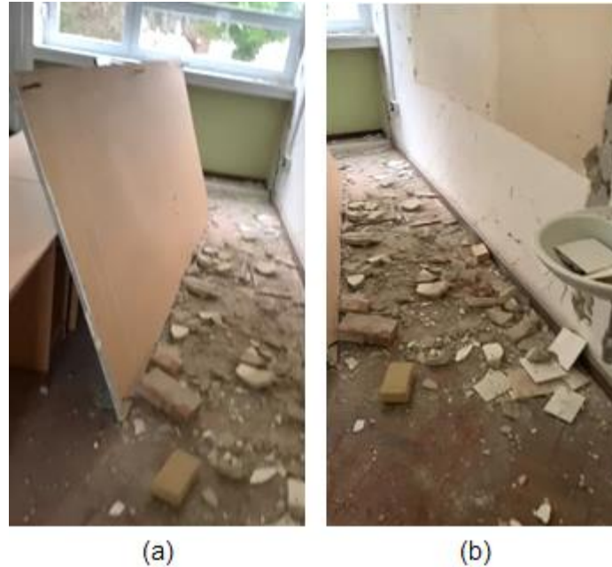
Figure 4.113. Detachment and collapse of the school board in one classroom (Faculty of Education - Učiteljski fakultet) (source: Marko Bartolac).
