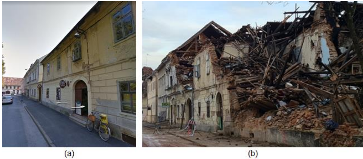
Figure 4.6. Collapsed URM buildings in downtown Petrinja (a) before the earthquake (source: Google Earth) and (b) after the earthquake (source: Nenad Bijelić).
