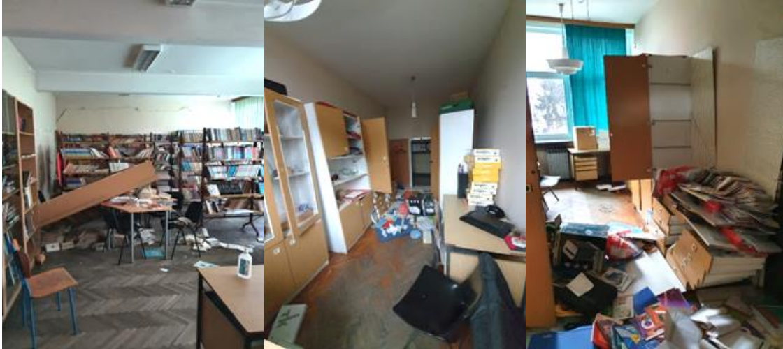
Figure 4.57. Items that fell off shelves and out of cabinets (source: Nenad Bijelić and Damir Lazarević).
