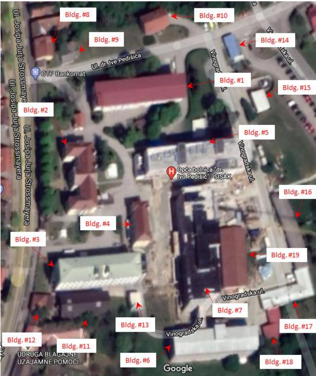
Figure 4.40. Plan view of the Dr. Ivo Pedišić General Hospital in Sisak. Buildings are enumerated for damage reporting purposes (source: Google Earth).
