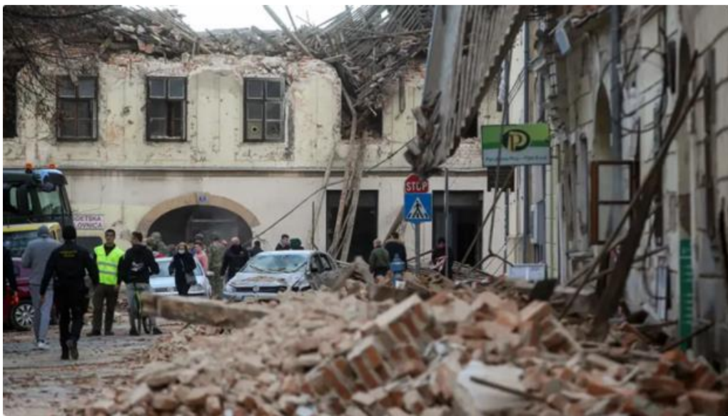
Figure 1.12. Croatian soldiers, firefighters, and residents next to heavily damaged buildings located in the center of Petrinja. Photo by Damir Senčar (Getty Images).
