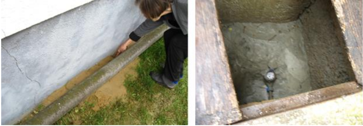
Figure 6.19. Liquefaction under a residential building with sandy soil ejected next to the structure and filling the underground space, Petrinja, Ulica Slavka Kolara (45.4349,16.2683, source Sonja Zlatović).
