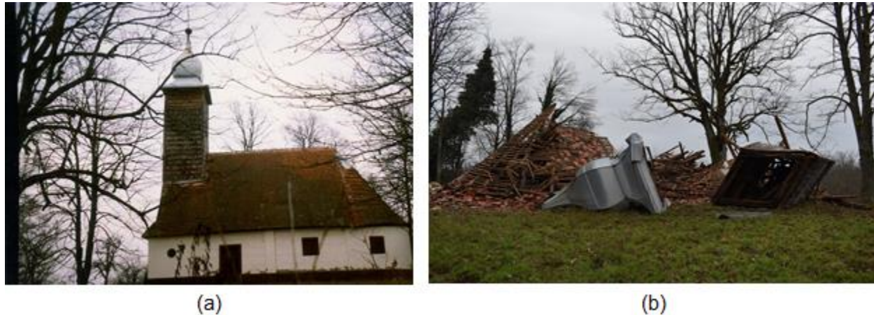
Figure 4.99. (a) Church in Majske Poljane (Hram Vaskrsenja Gospodnjeg) before the earthquake (source: Eparhija Gornjokarlovacka) and (b) Complete collapse of the Church (source: Eparhija Gornjokarlovacka).
