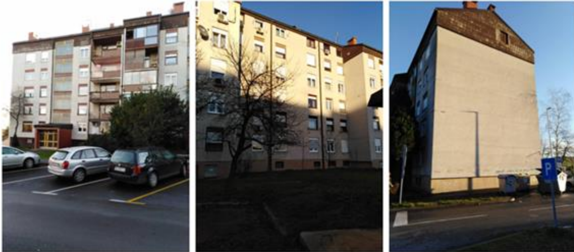
Figure 4.23. Buildings with RC structural walls that did not experience any damage, "Brzaj" settlement in Sisak (source: Maja Freiberger).
