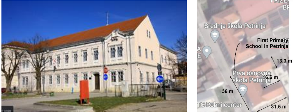
Figure 4.46. First Primary School in Petrinja: outside view before the earthquake (left) and U-shape plan view with dimensions (right) (source: Google Earth).
