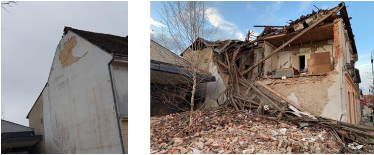
Figure 4.3. Typical wall and floor construction in older URM buildings, characterized by thick clay brick masonry walls, timber floors, and roofs. This building in Petrinja (adjacent to the KTC supermarket) was not significantly damaged in the December 28 M_w 5.2 earthquake but experienced gable wall and roof collapse in the December 29 M_w 6.4 earthquake (source: Joško Krolo).
