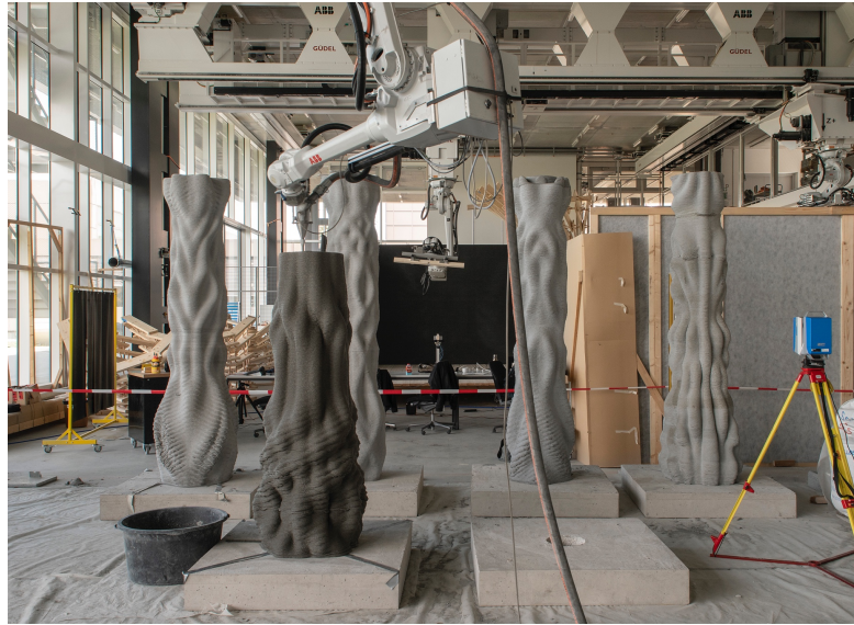
Figure 6.7: Fabrication of 2.7m high articulated columns, by layered extrusion, using a retarded OPC mortar and a CAC suspension as accelerator, with previously fabricated columns in the background for reference of process robustness (picture by Axel Crettenand). Fabrication time per column is approximately 2 hours, with all mortar coming from a single batch. At the time of placing, this mortar can self-support not more than 10cm.
