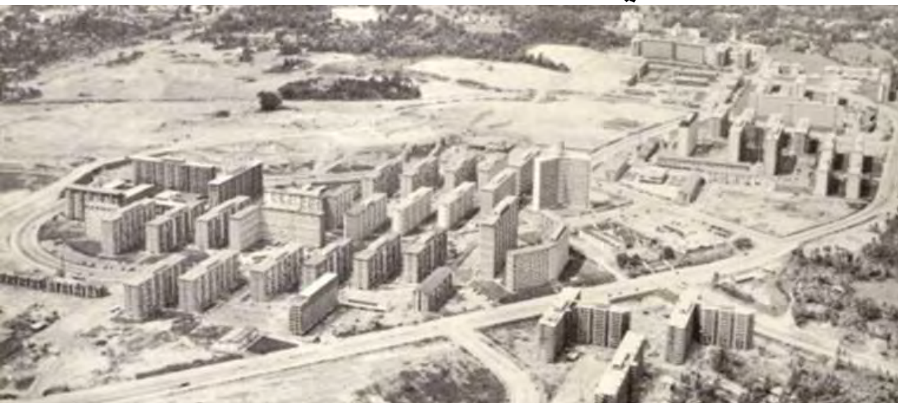
Figure 8.4 Beginning of construction in Toa Payoh in 1967 Source: (Heng, 2015)
