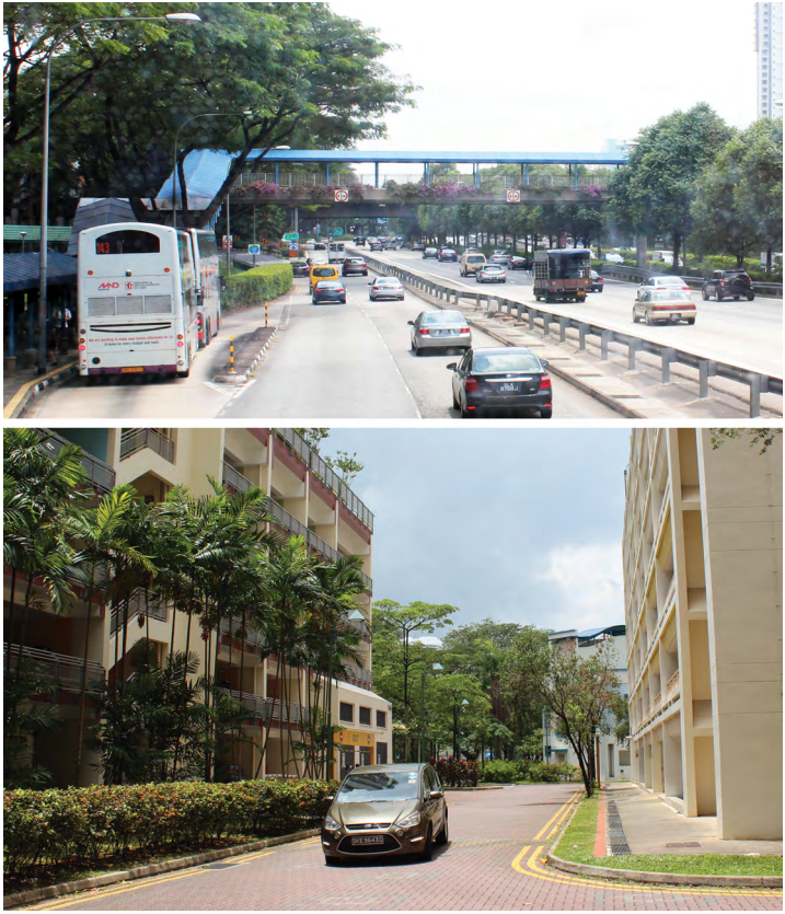
Figure 8.14 High traffic arterial roads (above) vs quieter internal roads (below)
