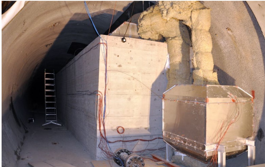
Figure 4: The heat storage in the pilot plant at Biasca.
