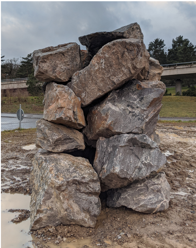
Fig. 9 Side elevation of constructed wall conveying double-faced structure and near-vertical orientation.
