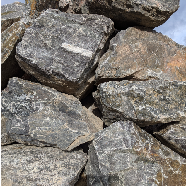
Fig. 5 Elevation detail of constructed wall. Rotationally invariant shape descriptors allow for a tight fit by initially matching available stone surfaces to corresponding negative geometry of the wall.
