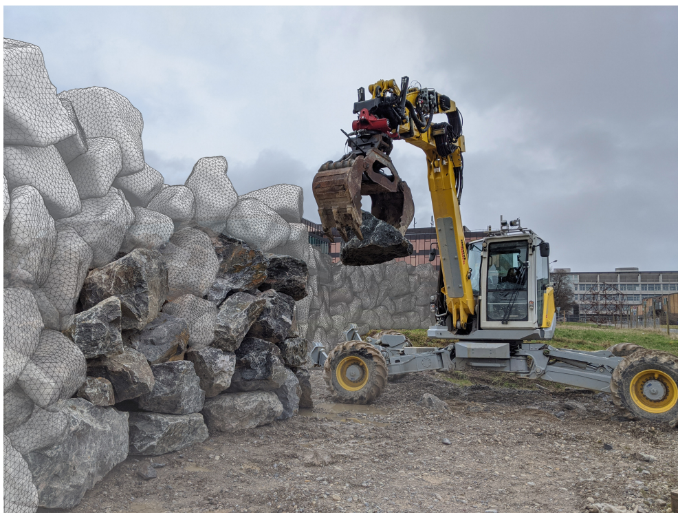
Fig. 11 In progress wall with overlay of potential extension of structure, generated by allowing the solver to continue with additional digital stone models.
