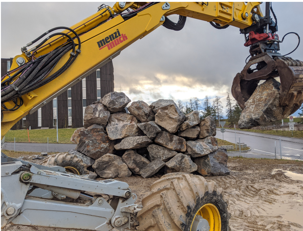
Fig. 1 Stone wall constructed with autonomous hydraulic excavator.
