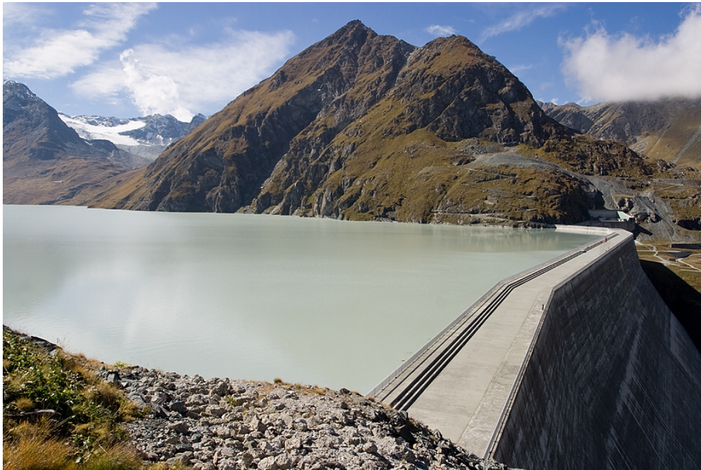
Fig. 1. Photo of the Grande Dixence Dam and Lac des Dix in Switzerland (Photo: Roland Zumbuehl, CC BY-SA 4.0)
