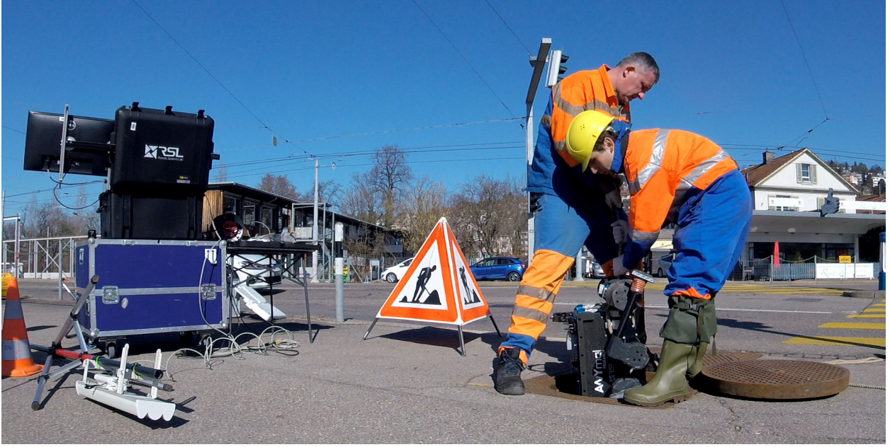
Figure 3: Depiction of the field test setup and the deployment of ANYmal into the sewer. The operator base station and warnings signs are visible in the background.
