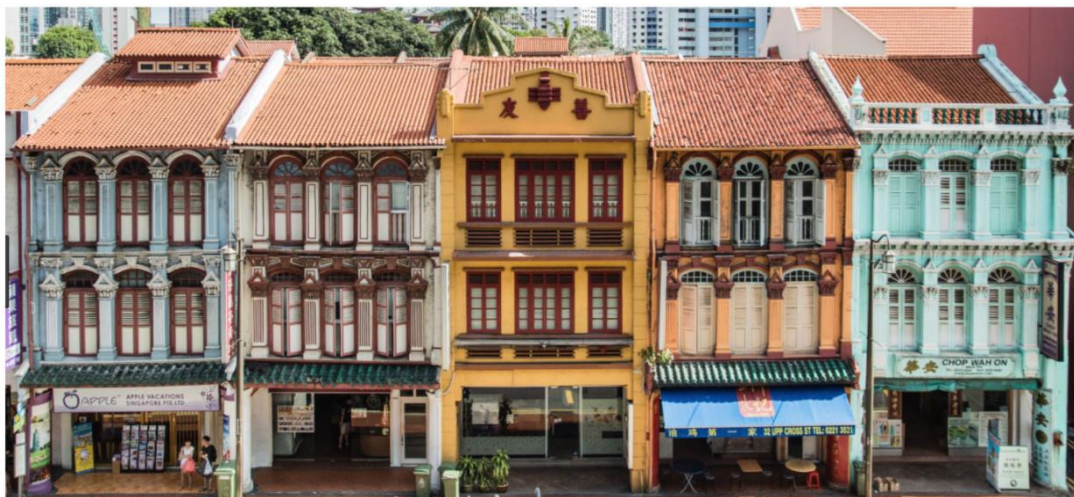
Figure 5-72. Traditional shop houses in Singapore’s Chinatown.
