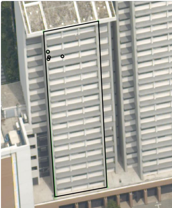
Figure 5-39. A facade full of windows. The four corners of a window are selected by the operator.
