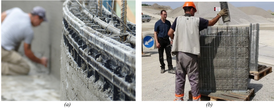
Fig. 5: Manually assembled stay-in-place formwork technologies: (a) Formatech's perforated plastic cages; (b) Coffra Suisse 3DR cages.
