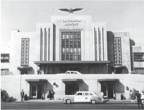
Figure 59: La Guardia Airport, Aldrich & Delano 1939, infamous steel eagle on terminal roof, photograph courtesy of Historic American Engineering Record, Library of Congress
