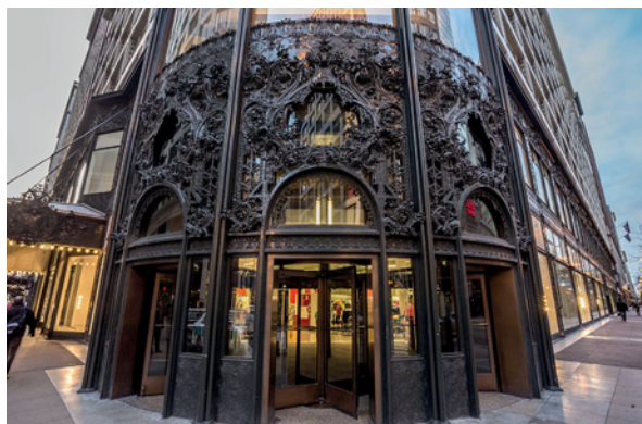
Figure 92: Carson Pirie Scott Building, Chicago, Illinois. Ca. 1900. Louis Sullivan, architect. Present day photograph by Chris Smith
